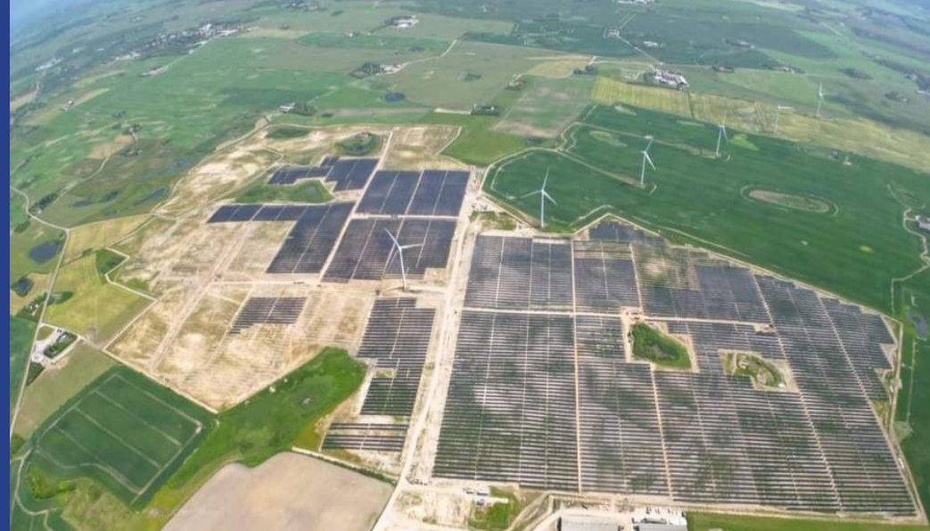
Lemvig Denmark 48MW , Tracker system Next Tracker
