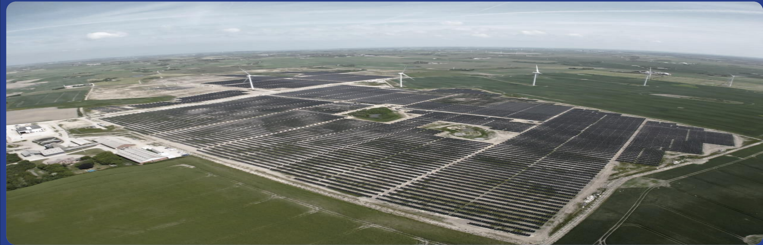
Lemvig Denmark 48MW , Tracker system Next Tracker
