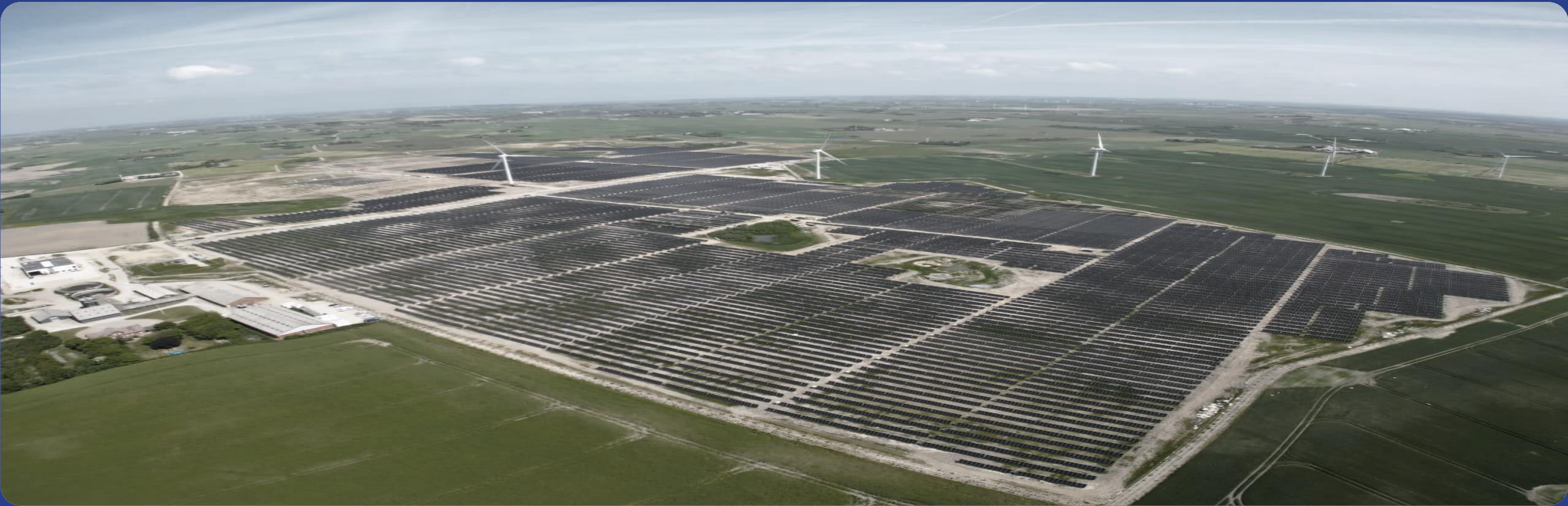
Lemvig Denmark 48MW , Tracker system Next Tracker
