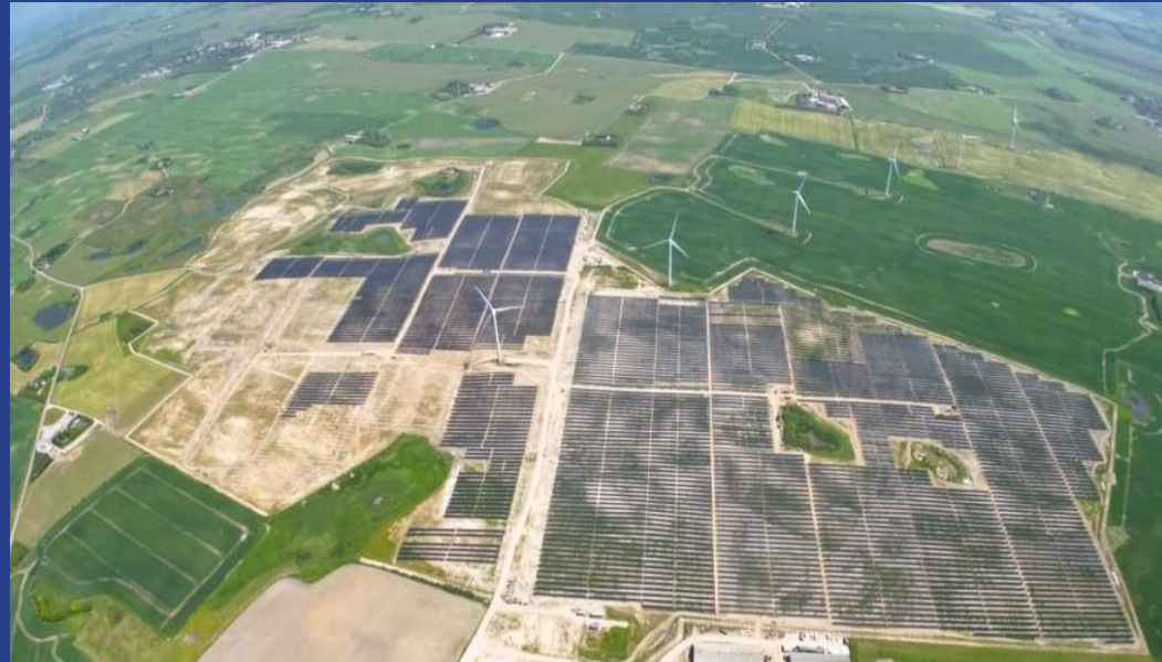
Lemvig Denmark 48MW , Tracker system Next Tracker
