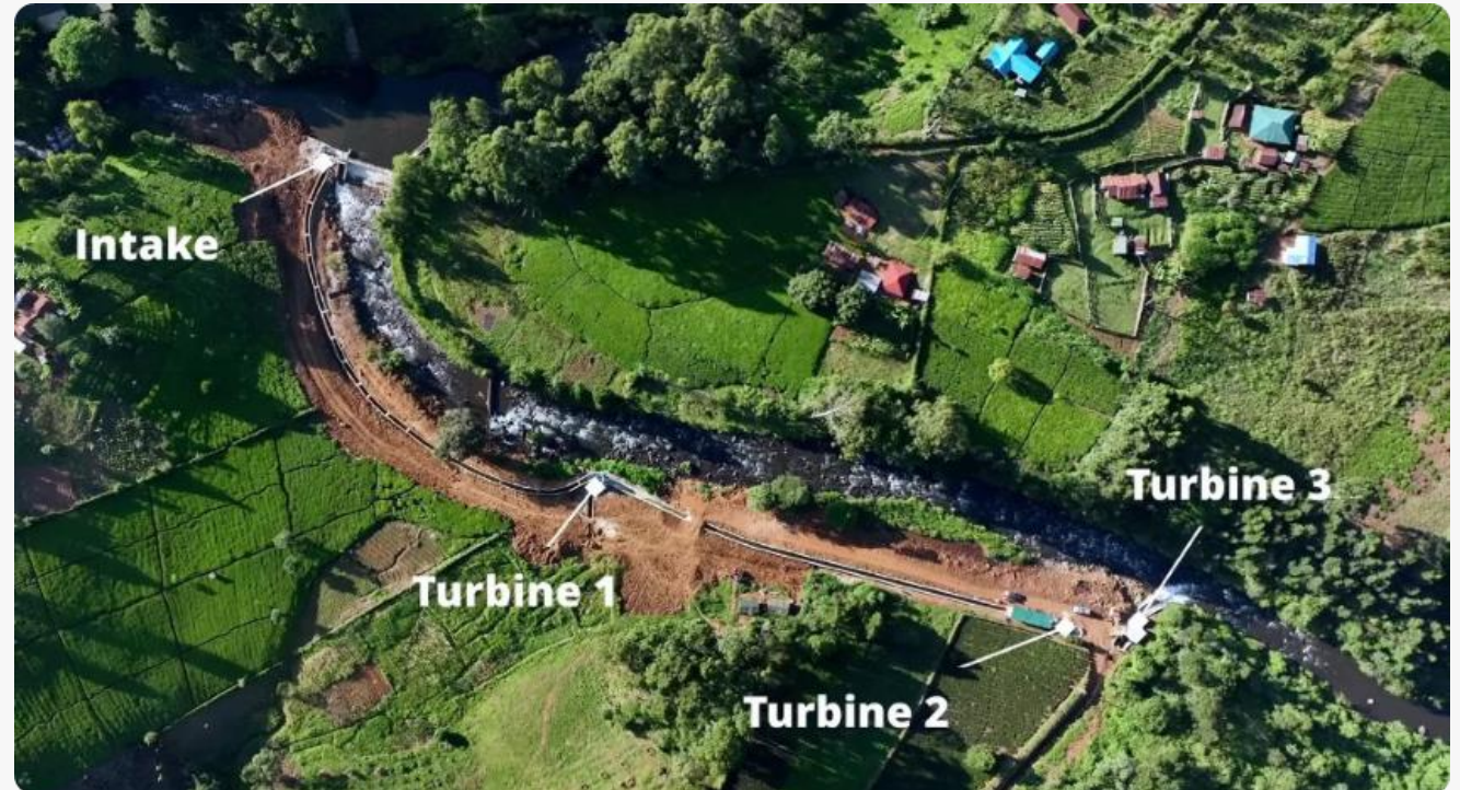
110kW project in Kenya
